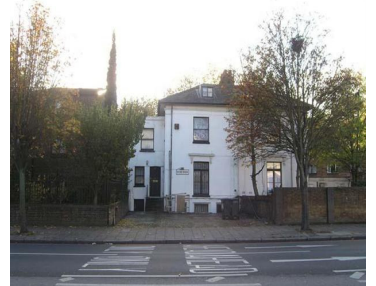
Lot 46 – Vacant House with planning for 5 flats
